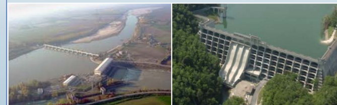
The Isola Serafini weir crossing the Po River (left) and the Molato concrete buttress dam (right)
