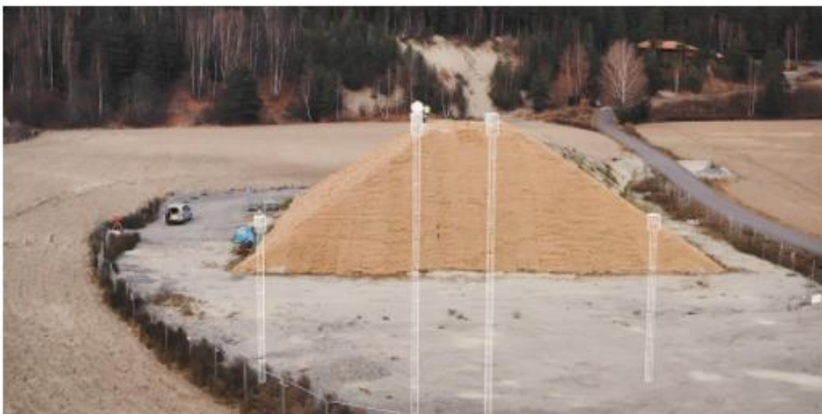
Figure 91 Full-scale testing of a fill in a geo-test site in Norway
