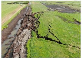
Figure 1. Recent failure of a dyke founded on organic soils
